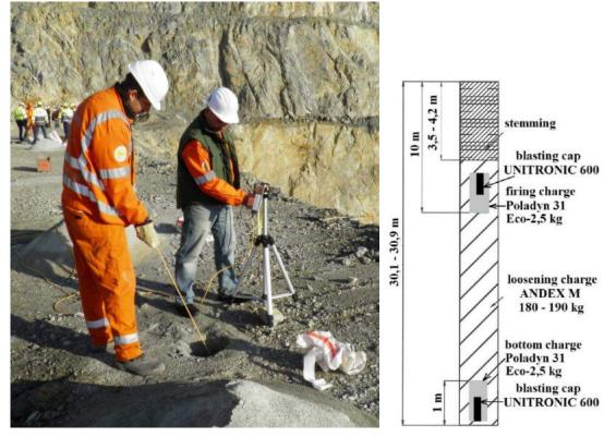
Figure 5. Charging, incklinometer measuring of boreholes and construction of charges No. 693 - 698 at the III. etage of the quarry Trebejov.
